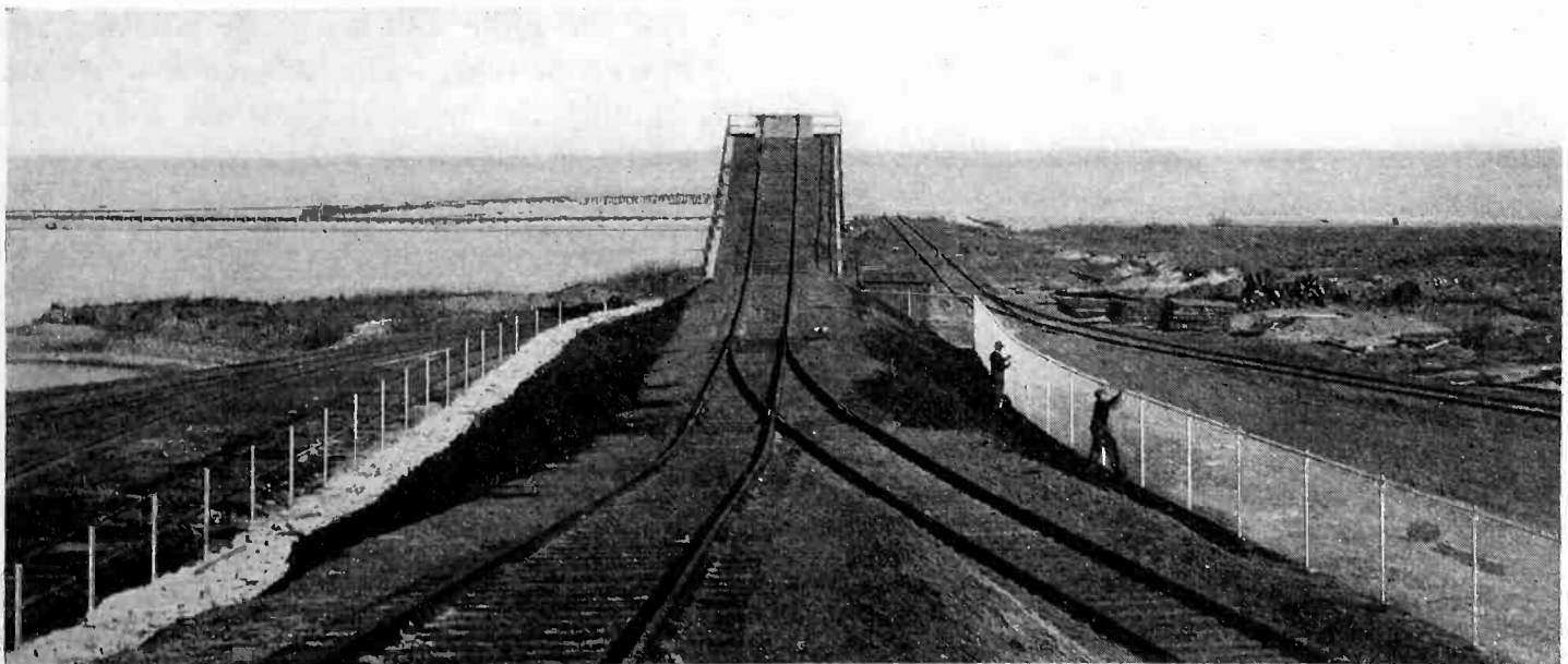
In this car-dumping installation at Waukegan, Ill., as the empty car travels down the return track, it cuts off a beam of light, causing the relay to ring the bell in the operator's cab. The bell warns him that the car has reached the predetermined point and that the car-retarding mechanism should be operated
